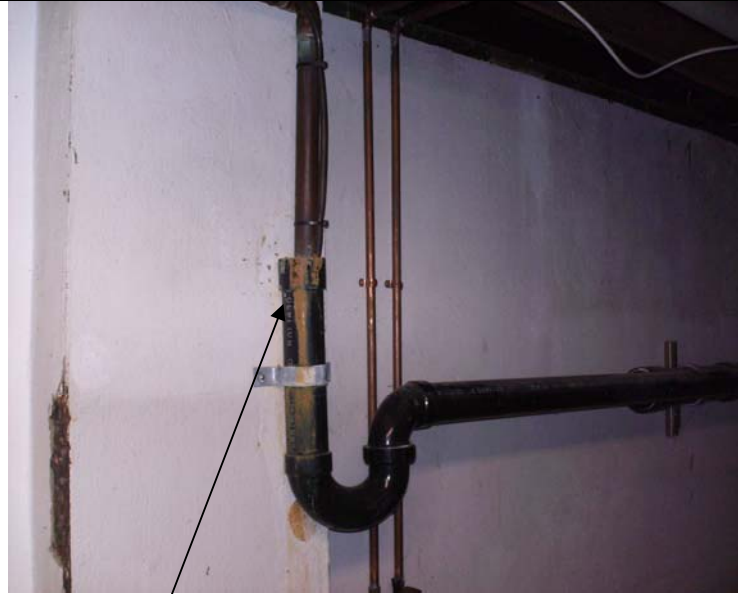
The basement sump pump discharges into the sewer. This is improper. The sump should discharge to the exterior of the home.
