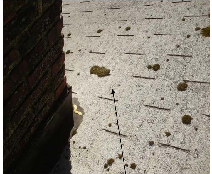
We recommend replacing the worn deteriorated roof shingles.
