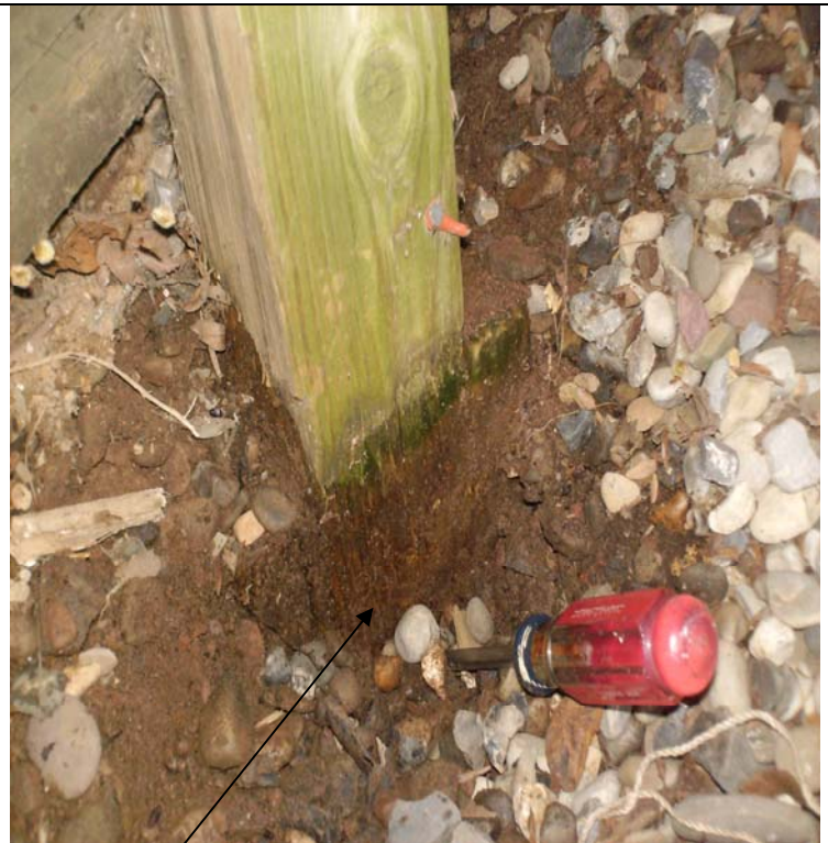
Install proper footings for the deck support posts.
