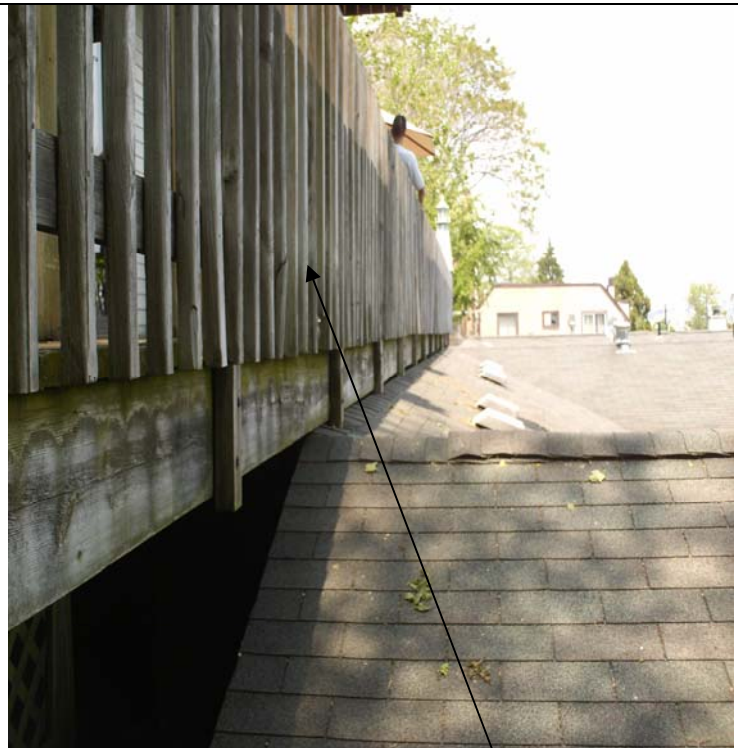
Secure the loose rear deck safety railing.
