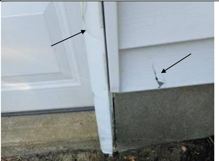
Damaged vinyl siding along garage. Also dented garage door jamb aluminum capping.
